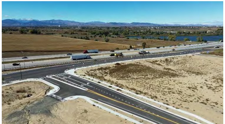
I25 Frontage Road and Colleen Street Improvements
