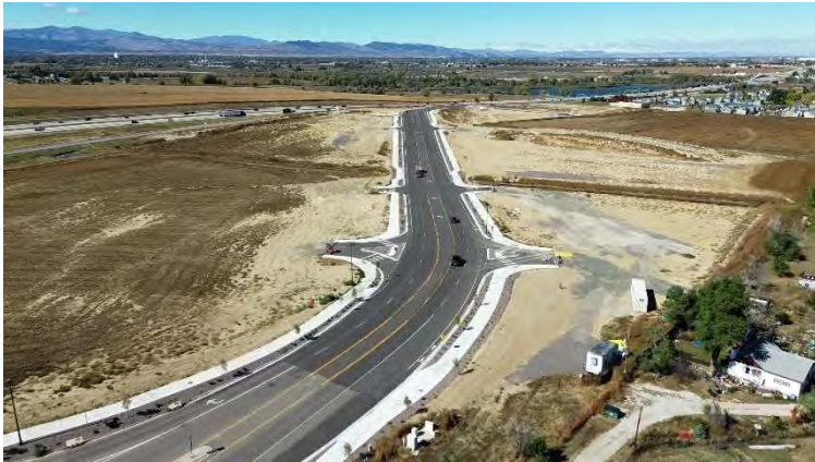
Overall View – Facing Northwest
