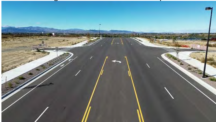
I25 Frontage Road Improvements – Facing Northwest
