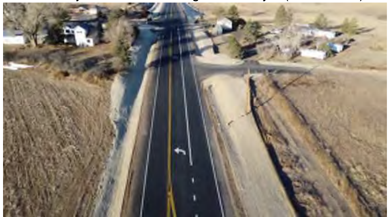
E County Rd 18 (View: West)
