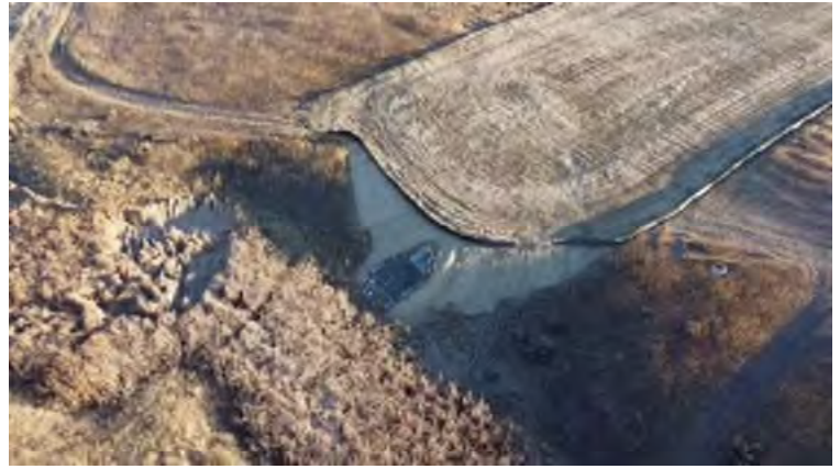
Multi-Family Offsite Storm Line 1 Outfall – (View: South)
