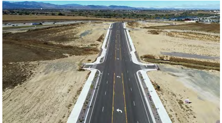
I25 Frontage Road Improvements – Facing Northwest
