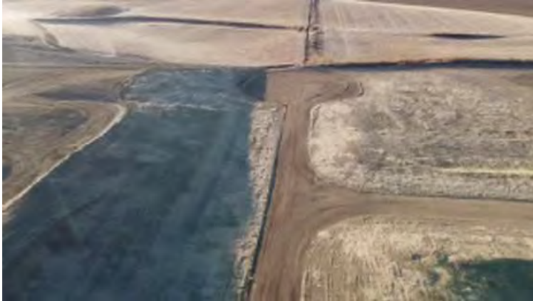
Elsie Ave and Caliber Pkwy – (View: South)
