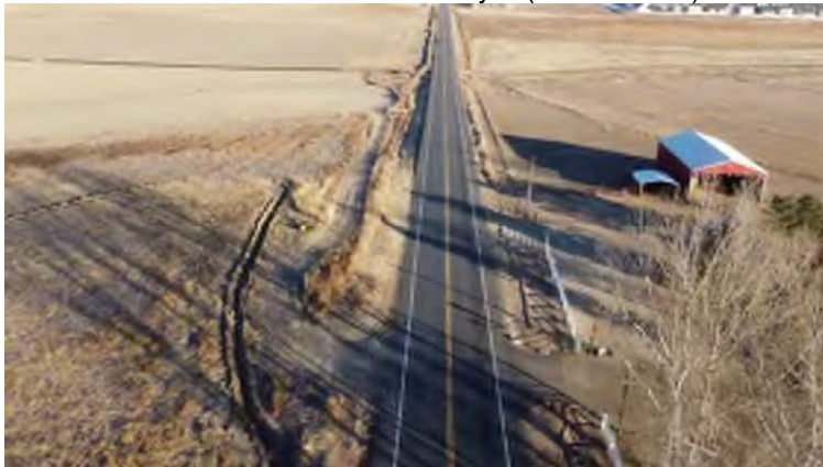
S County Rd 3E North of E CO Rd 16 – (View: North)
