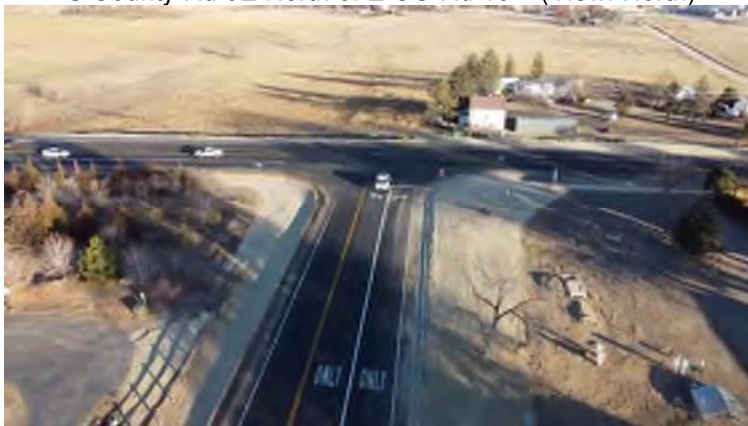
S County Rd 3E and E County Rd 18 (View: North)
