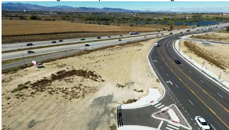
Earthwork Improvements – Facing Northwest
