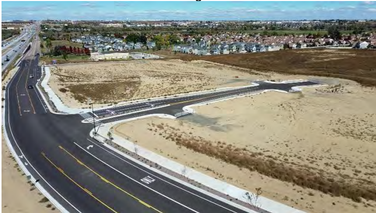
I25 Frontage Road and Colleen Street Improvements
