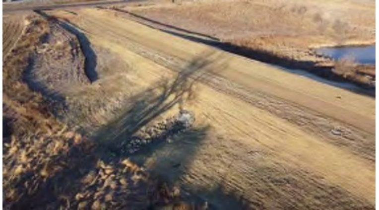
Multi-Family Offsite Storm Line 2 Inlet – (View: Northwest)
