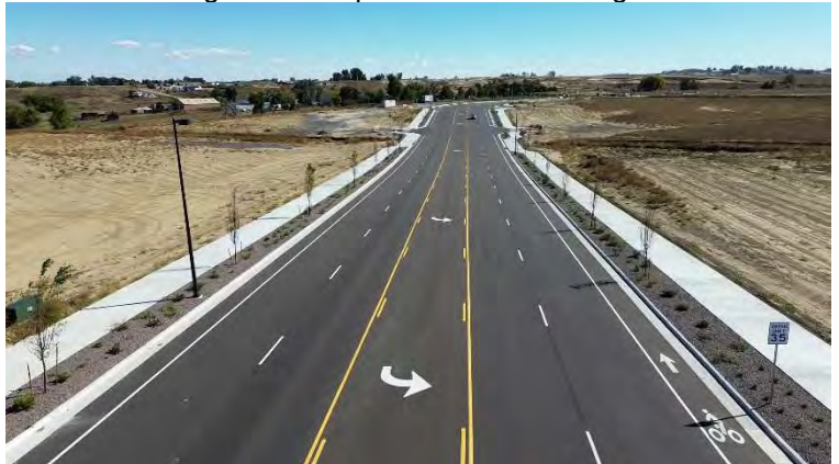
I25 Frontage Road Improvements – Facing Southeast
