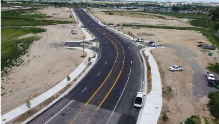
Frontage Road – Facing Northwest - STA.103+00
