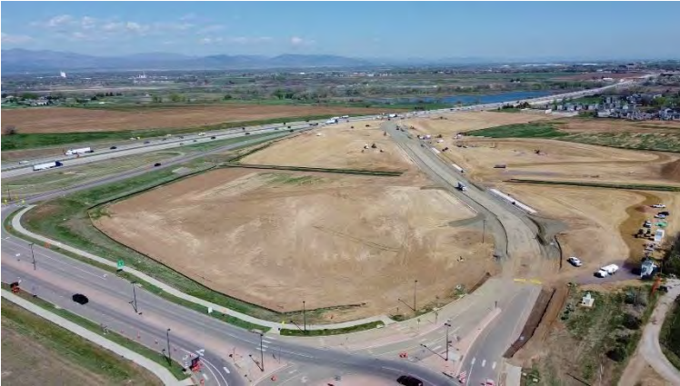
Overall View – Facing Northwest
