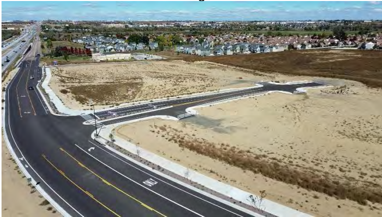
I25 Frontage Road and Colleen Street Improvements
