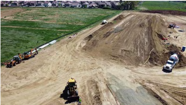
Earthwork in Tract B – Facing East
