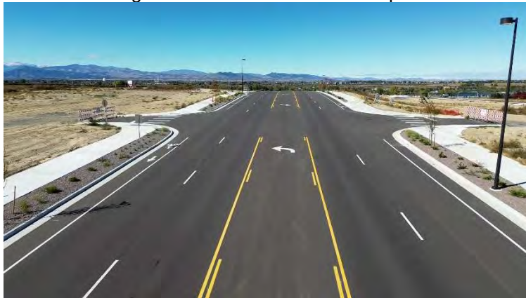
I25 Frontage Road Improvements – Facing Northwest
