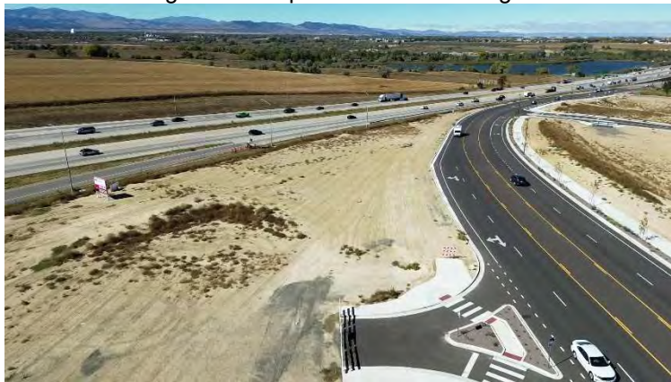
Earthwork Improvements – Facing Northwest
