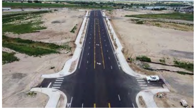
Frontage Road – Facing Northwest - STA.107+50
