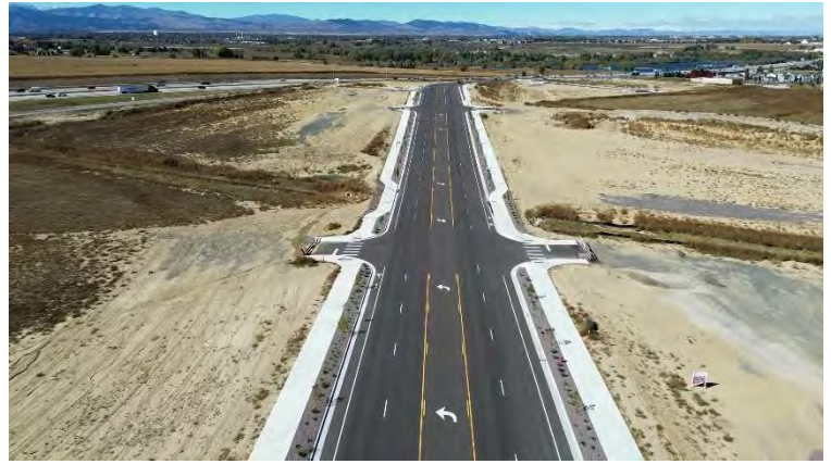
I25 Frontage Road Improvements – Facing Northwest
