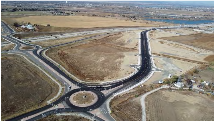
Overall – (View: Northwest)
