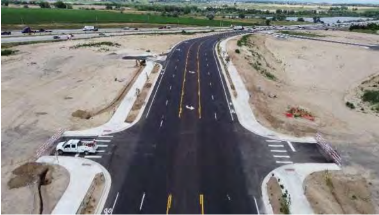
Frontage Road – Facing Northwest - STA.113+00
