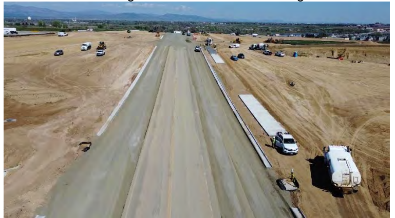
Frontage Road Work – Facing Northwest
