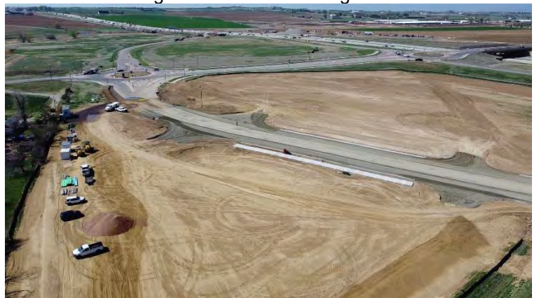
Southern Portion of Site – Facing Southwest
