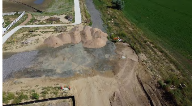
Offsite Sanitary Sewer View: North
