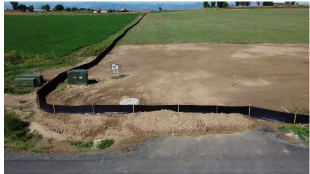
Offsite Sanitary Sewer View: West
