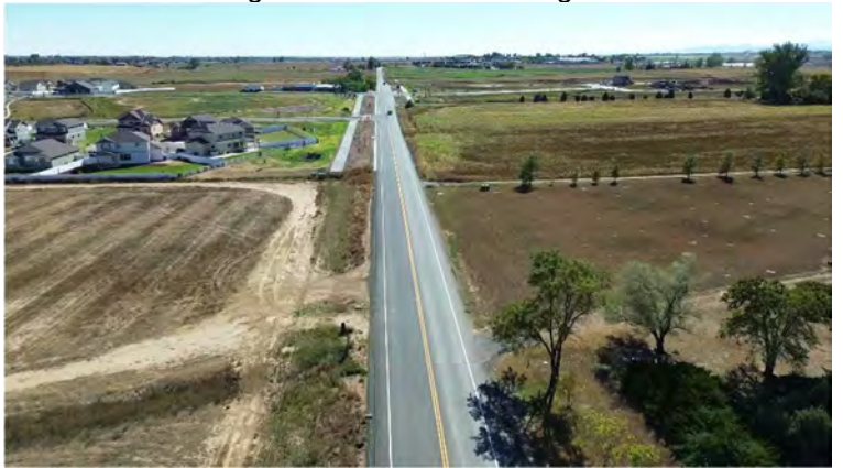
CR 3E Street Improvements – Facing South
