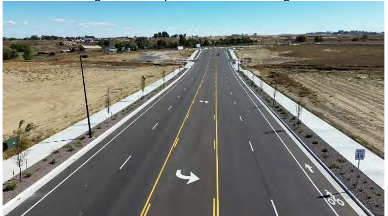
I25 Frontage Road Improvements – Facing Southeast
