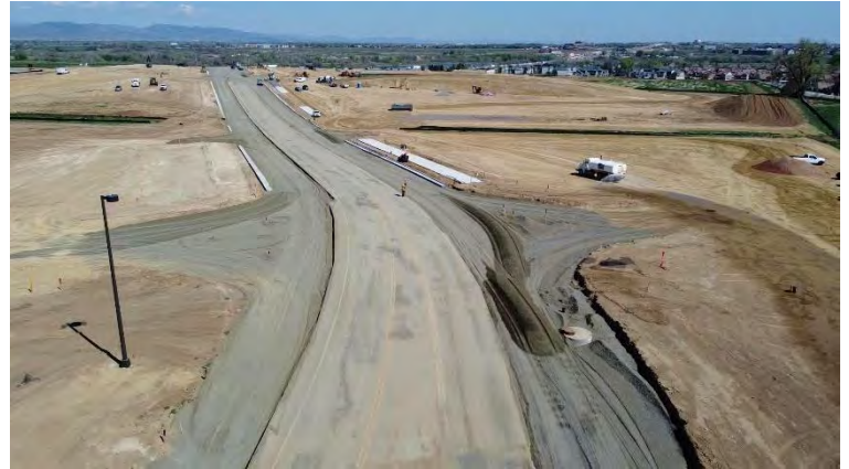
Frontage Road Work – Facing Northwest
