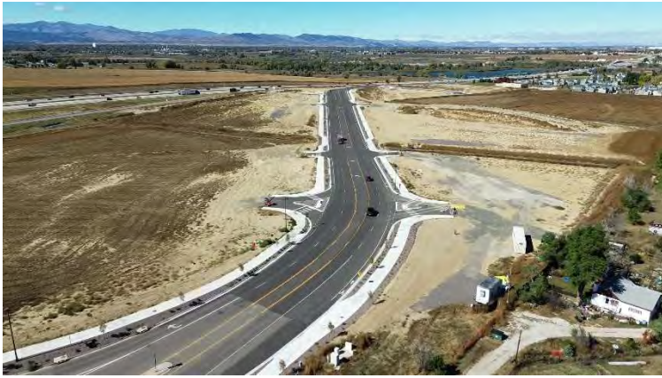
Overall View – Facing Northwest
