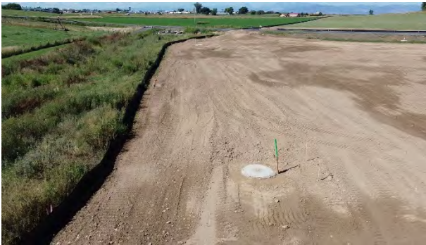
Offsite Sanitary Sewer View: Southwest
