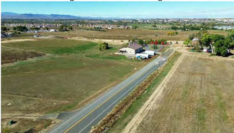
CR 3E Street Improvements – Facing Northwest
