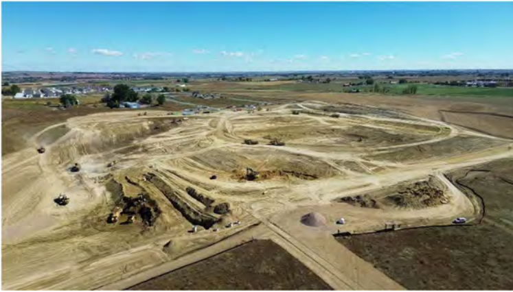
Filing 3 Overall View – Facing Southeast
