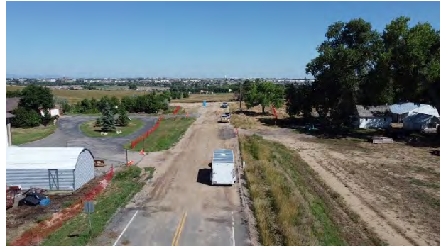
County Road 3E View: North
