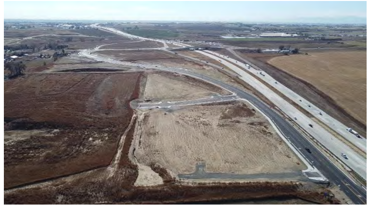
Overall – (View: South)
