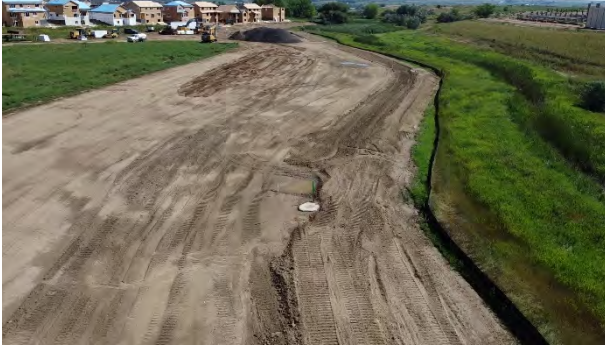
Offsite Sanitary Sewer View: Northeast
