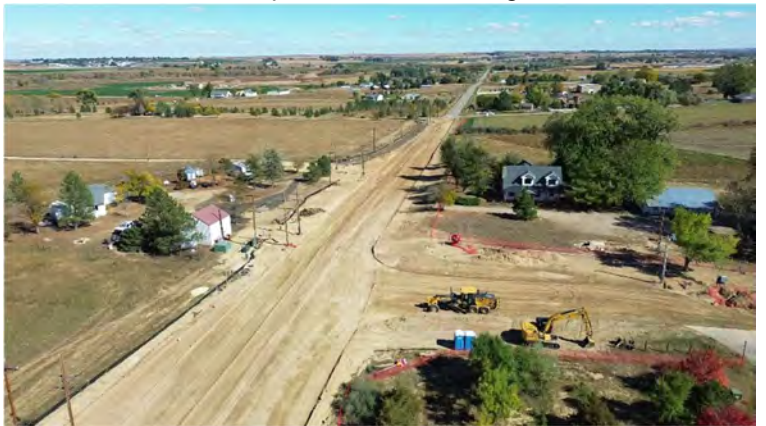
CR 3E Street Improvements – Facing East
