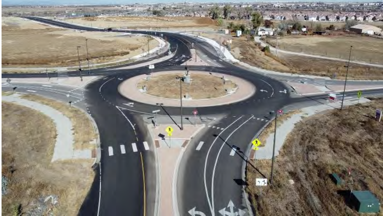
E County Rd 18 & I25 Frontage Road – (View: North)
