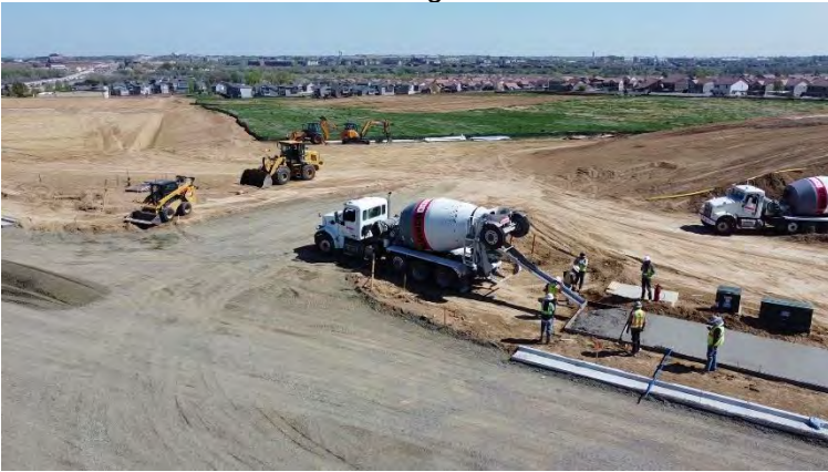
Frontage Road Work – Facing Northeast
