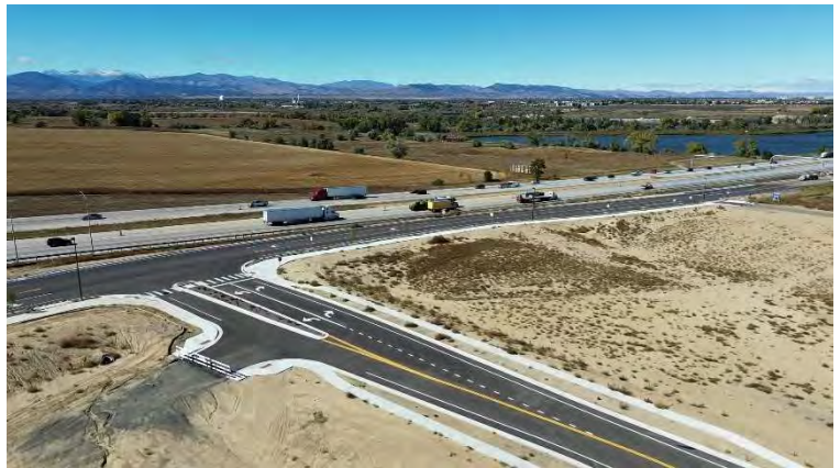
I25 Frontage Road and Colleen Street Improvements
