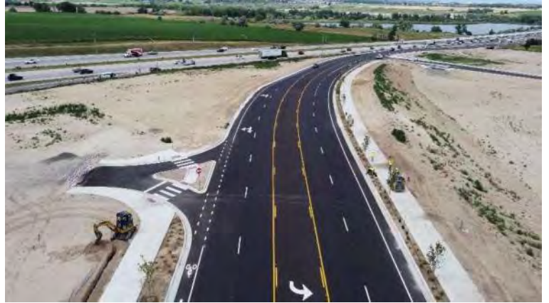
Frontage Road – Facing Northwest - STA.116+00
