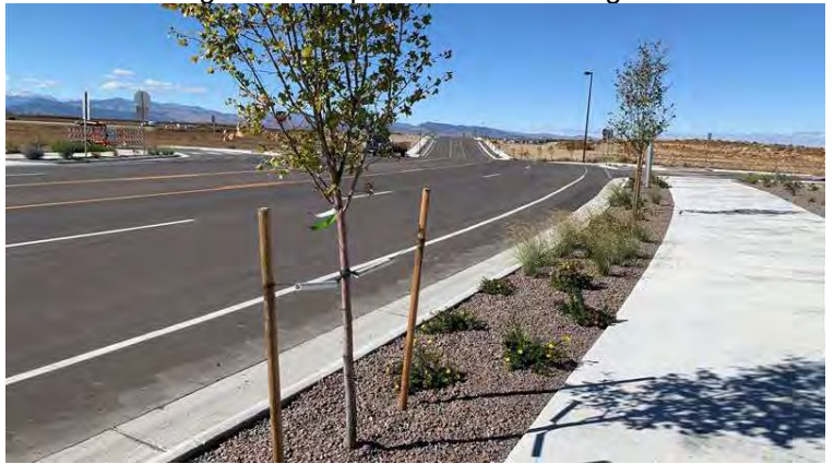
Landscape Improvements along I25 Frontage Road
