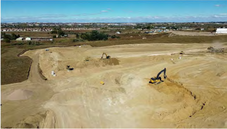
Filing 3 Overall View – Facing Northeast
