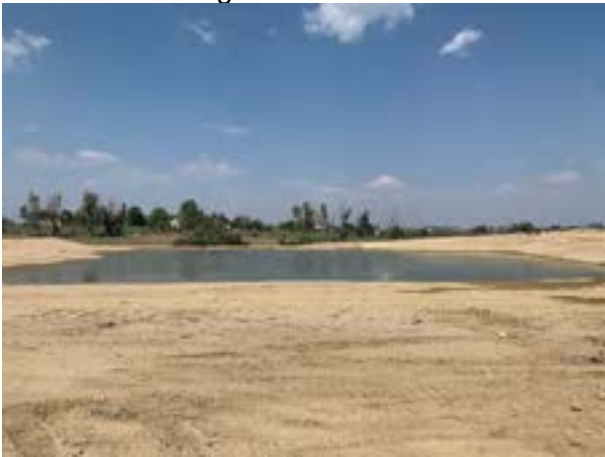
Filing 1 – Detention Pond
