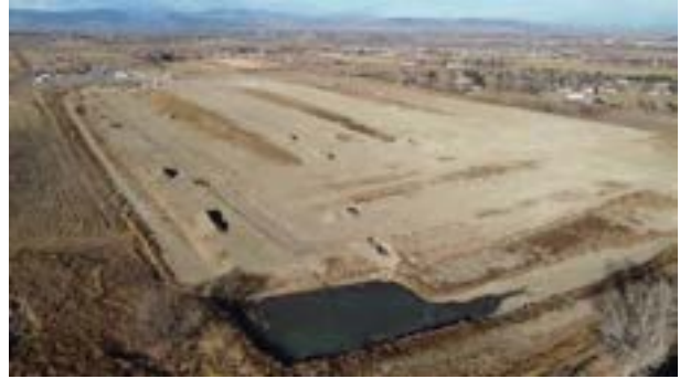
Area A facing NW
