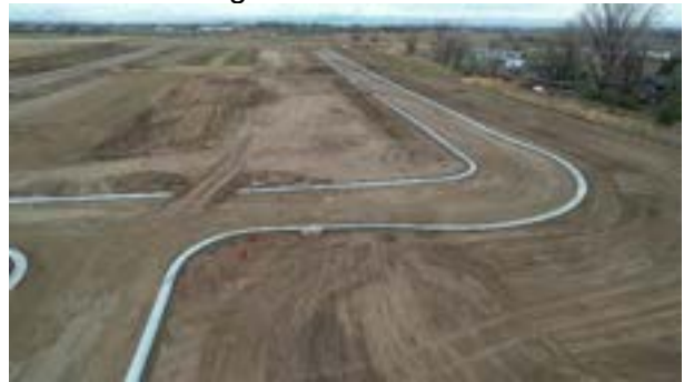
Curb Improvements in Filing 1
