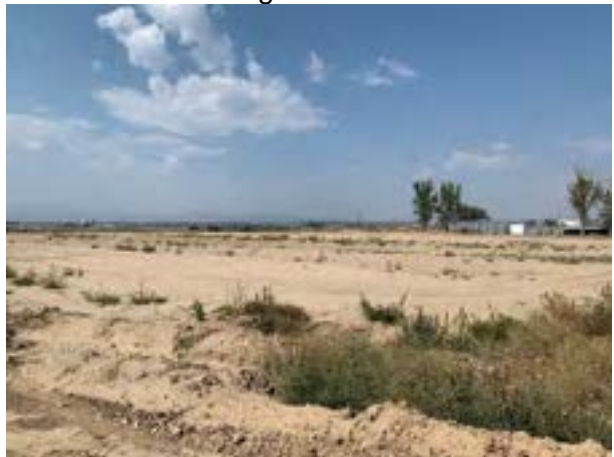
Filing 2 – Detention Pond
