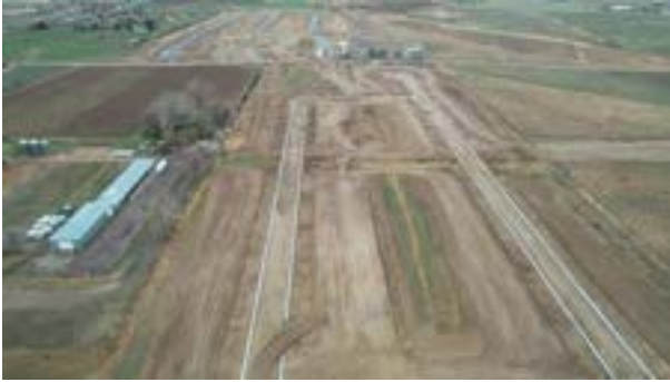
Filing 2 – Street Grading & Concrete
