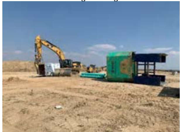
Filing 1 – Trench Box
