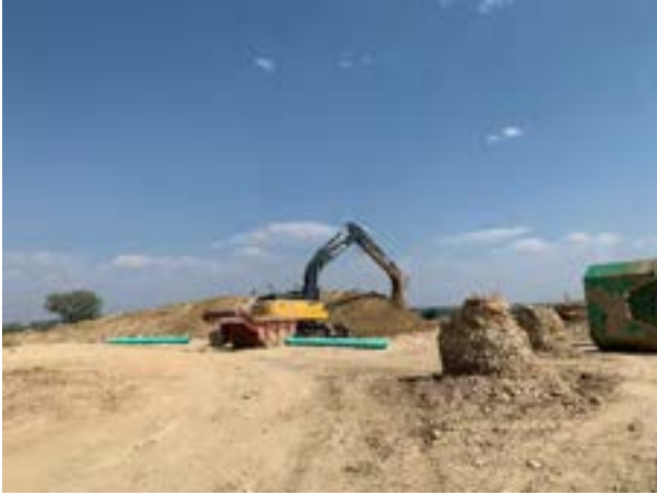
Filing 1 – Sewer Line
