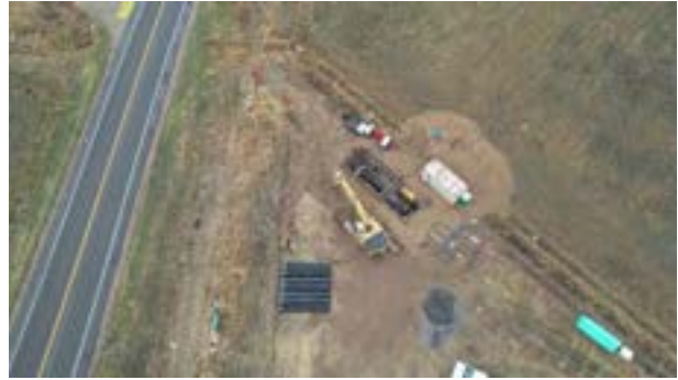
North Ridge Water Improvements
