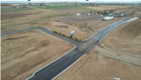
Fine Grading Crew on Site
