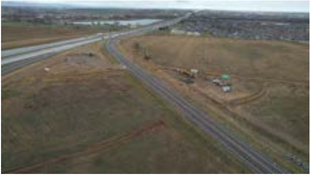
North Ridge Water Improvements
